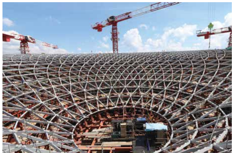
Close to 18,000 pieces of steel element and over 6,000 steel nodes were used in the construction of the Jewel façade.
