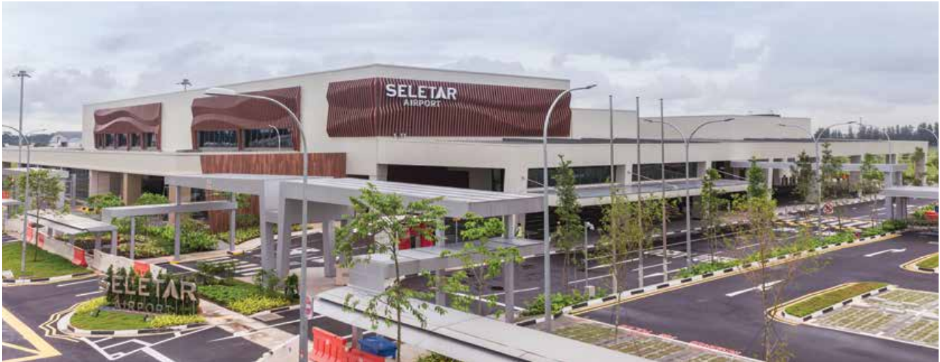
▶ Seletar Airport's new passenger terminal building is designed to handle 700,000 passenger movements annually.
